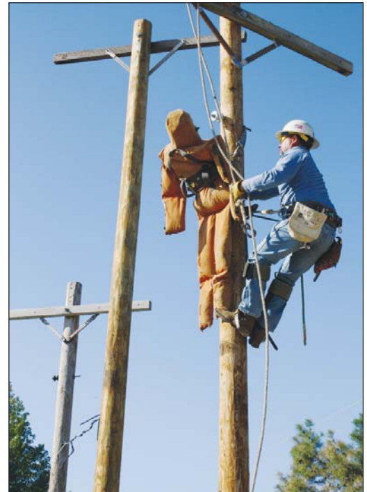
Allen Hare performing pole top rescue
